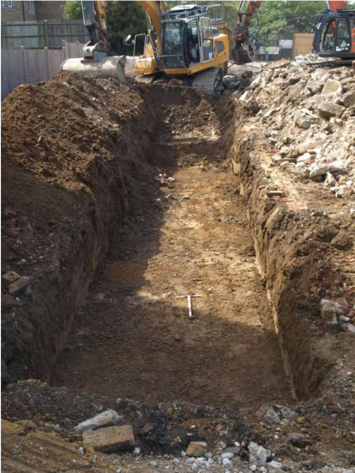
Plate 4: Evaluation Trench 2 looking south-west. The wall of recently demolished building visible alongside to the right. Half and point three metre scales.
